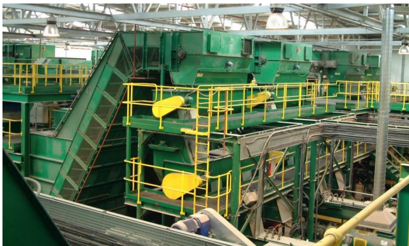
A fuel production plant built by ART in 2003 – processing 230,000 tonnes a year of wastes with no atmospheric emissions.
